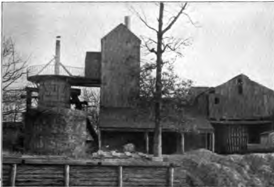
FIG. 2.—MUIRKIRK FURNACE, MUIRKIRK, PRINCE GEORGE'S COUNTY.
